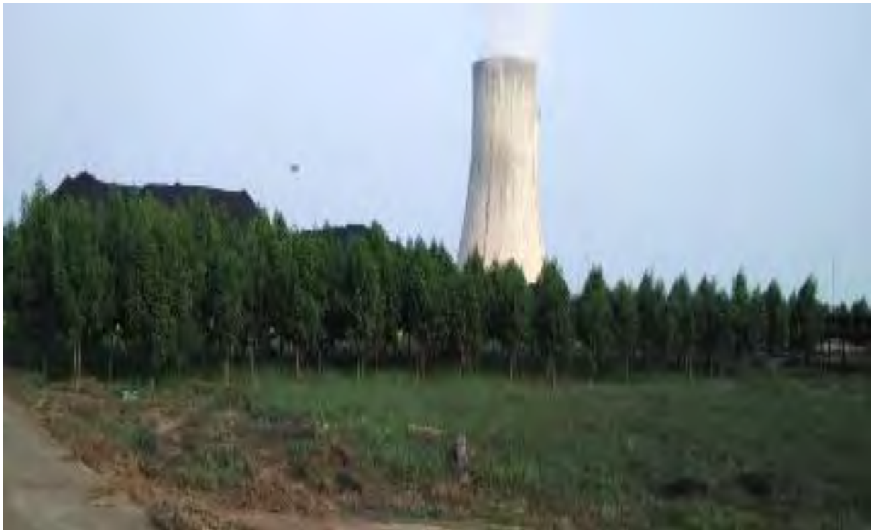
WIND BREAK PLANTATION AROUND COAL YARD
