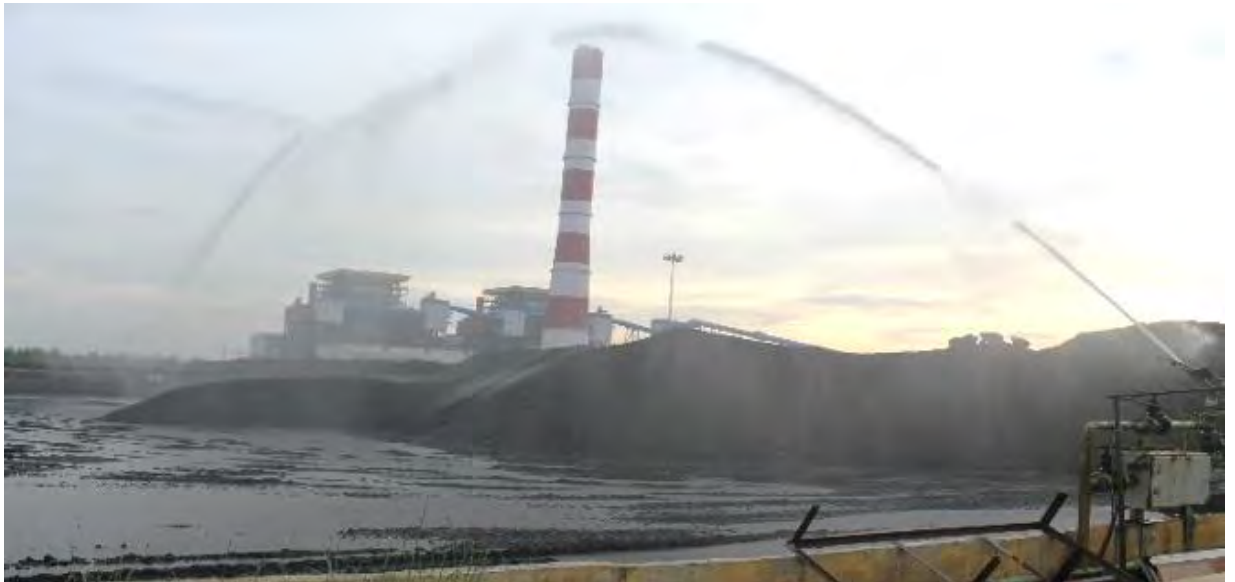
COAL YARD WATER SPRINKLING
