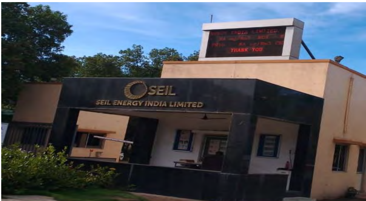
MAIN GATE DISPLAY BOARD - AMBIENT AIR QUALITY & EMISSIONS DATA DISPLAY
