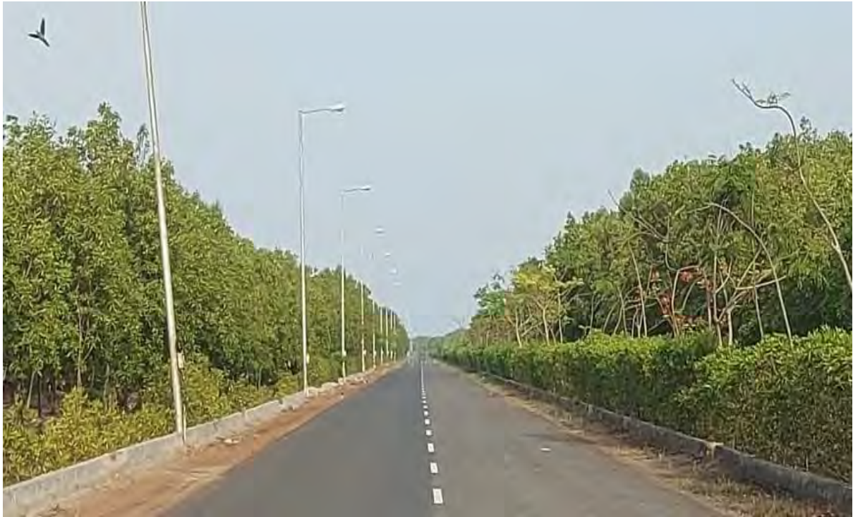
GREEN COVER ALONG PIPE RACK & INTERNAL ROADS
