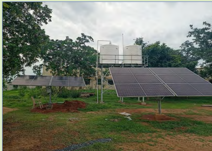
Solar Pump installation at Plantation Site
